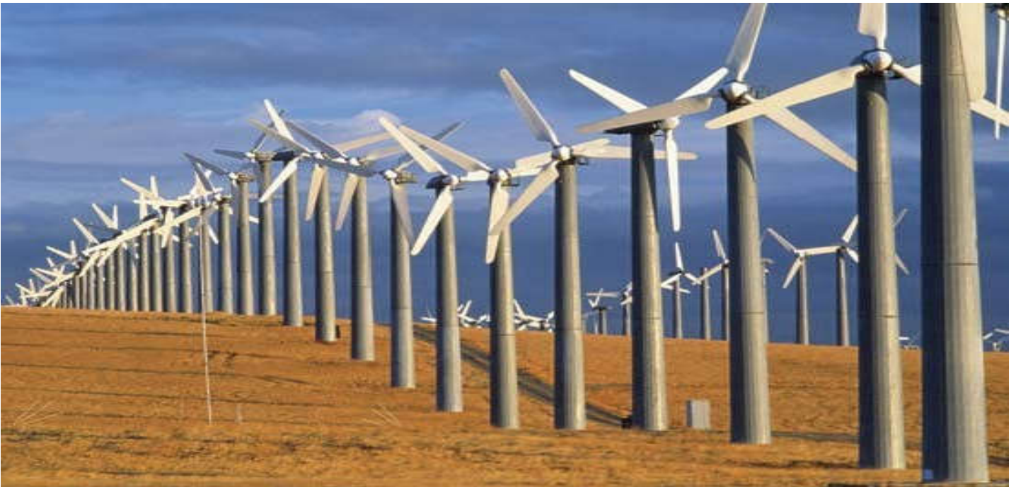
Figure 1 - Wind turbines in Tracy, Calif.
